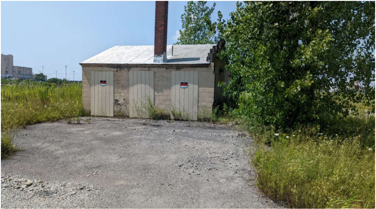
Photo #7: Abandoned building (viewing east wall)
