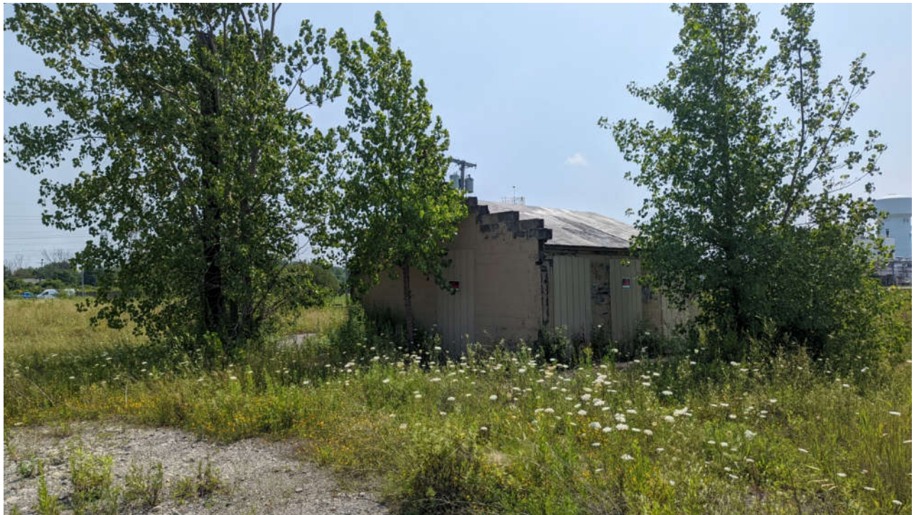
Photo #8: Abandoned building (viewing northwest corner)
