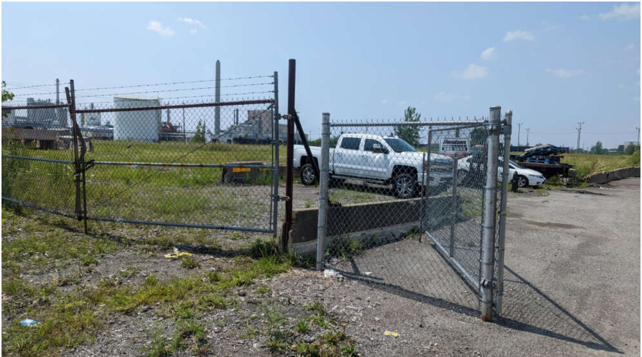
Photo #3: At gate on Simmons looking southwest into site
